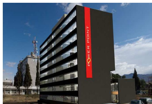
EuroPoint Office Building
